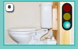
Since many close coupled WC suites do not have the space between the WC pan spigot and the wall, you may have to batten the cistern off the wall to make room for the Saniflo. However Sanislim will fit behind most closed coupled WC suites without the need for this.
