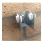
Wall Brackets — Offer up the radiator in the desired position, mark the bracket positions and fixing holes. The radiator should be placed a minimum of 10cm from the floor. Using the appropriate drill and fixings attach the brackets to the wall. After installing the plastic inserts into the hook part of the bracket the radiator can then be hung from the brackets
