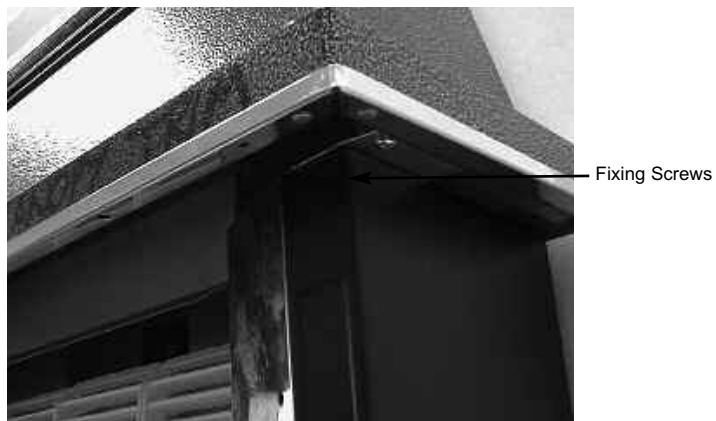
Fig. 7 Removing the Upper Outer Case Fixing Screws
