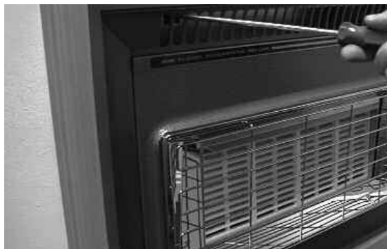
Fig. 10 Removing the Upper Outer Case Fixing Screws
