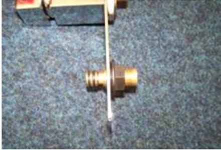
Fit the rubber washer and screw the backnut up to it from behind the plate.
