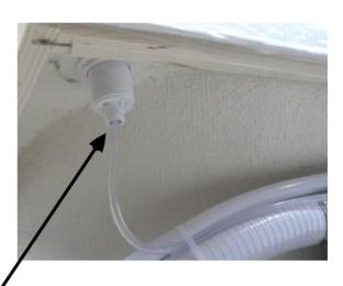
Check Capillary pipe is attached to on/off button and pump
